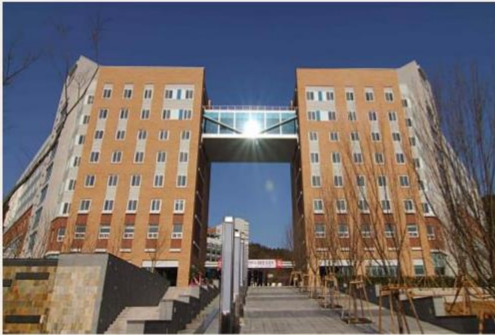
Panoramic view of Hoyeon Dormitory
